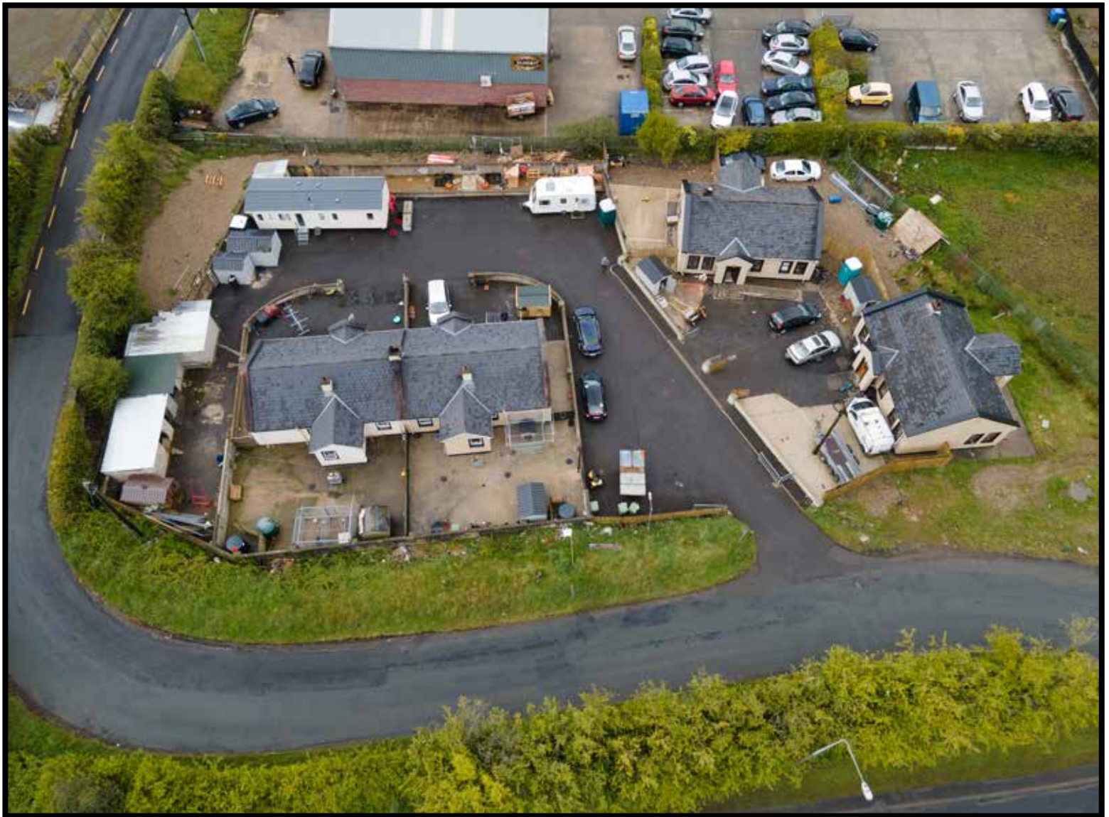
Cullion Road Group Housing Scheme
